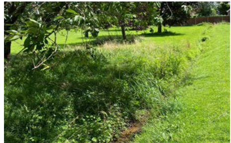
Drainage ditch in public open space
