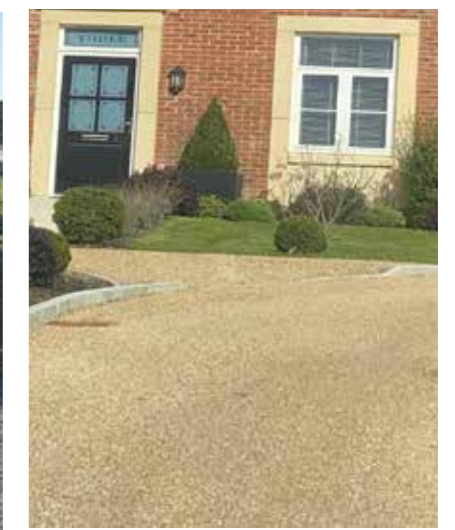
Golden aggregate to secondary roads and driveways
